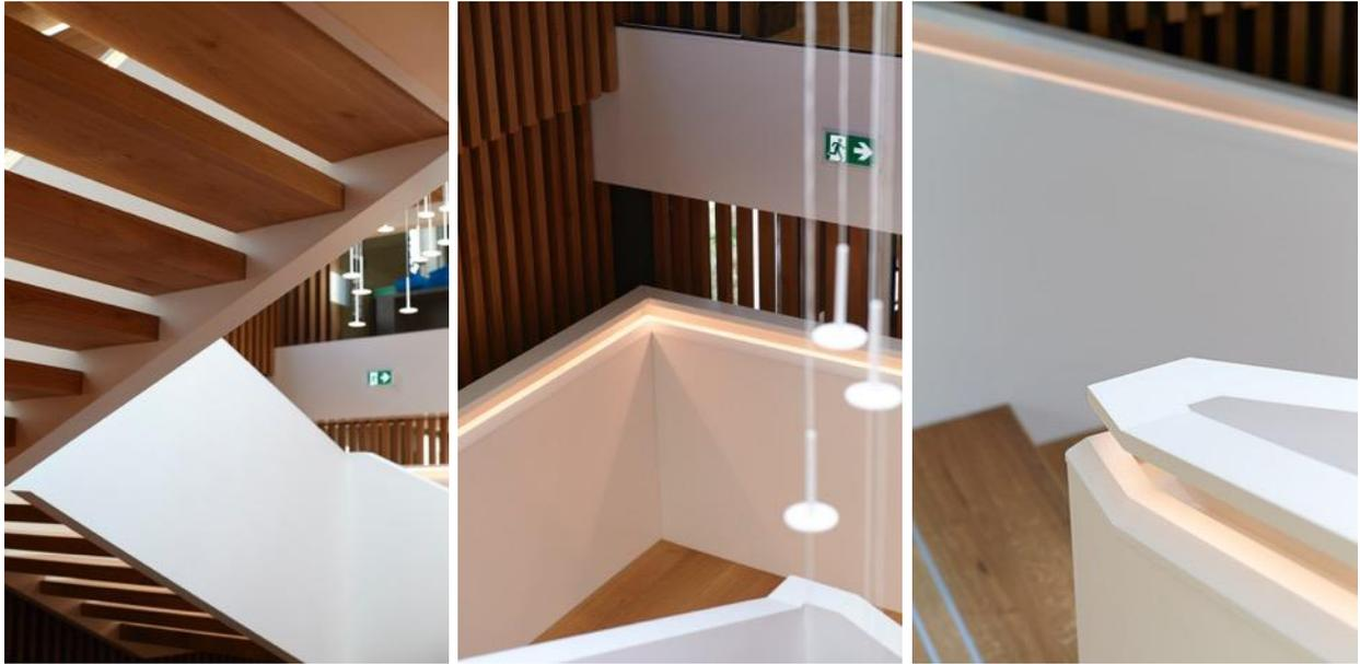
Further enhancing the wood, the railings installed all along the path of this atrium structure – with the exception of the landings – are clad with 12-mm bonded, seamless HI-MACS® Alpine White panels, on top of a metal structure with a slightly beveled lip.
