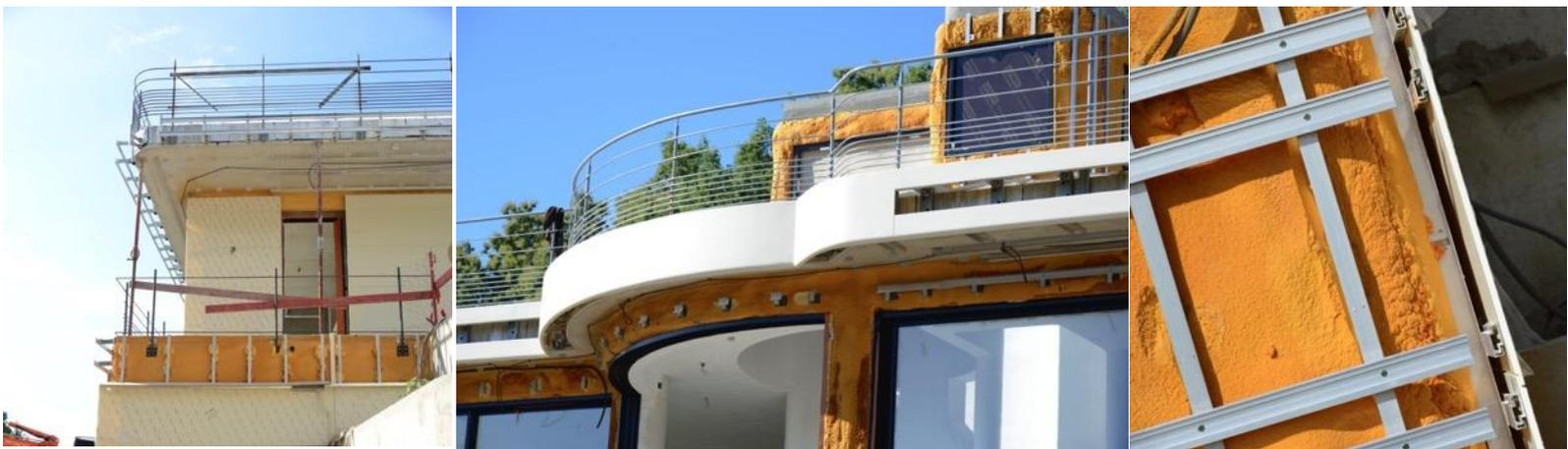
With a surface area of 550 m<sup>2</sup>, the façade is composed of a primary BWM 100 metal framework placed over the raw concrete façade, covered and insulated with polyurethane foam, into which 220 12-mm-thick **HI-MACS®** Cream panels are fitted using Keil sleeve anchors that are invisible from the exterior. The thermoformed panels follow the curves, pillars and porthole windows of the villa perfectly, collectively forming an outer facing in line with expectations.
