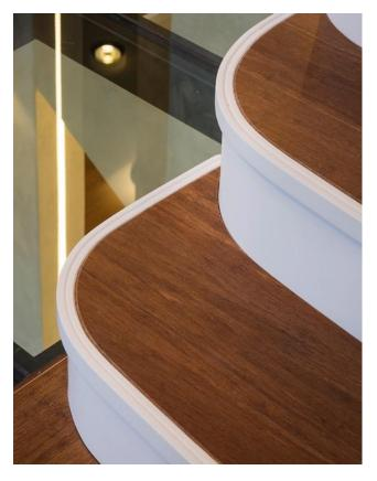
The risers and nosings on the stairways to each level, made of **HI-MACS**®, are coupled with a type of bamboo laminate hewn on-site. This use of wood, combined with the purity of the Solid Surface, imbues the entire staircase (jointly created by Menuiserie Bareau and SARL Acorrs) with fluidity and warmth.
