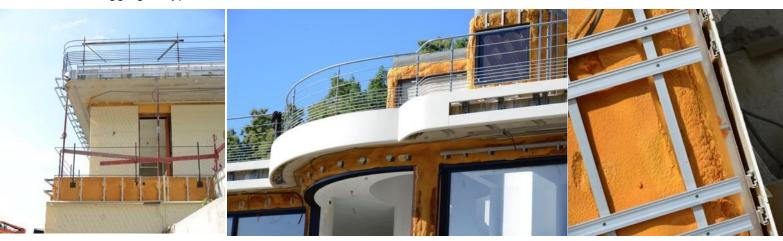
With a surface area of 550 m², the façade is composed of a primary BWM 100 metal framework placed over the raw concrete façade, covered and insulated with polyurethane foam, into which 220 12-mm-thick **HI-MACS®** Cream panels are fitted using Keil sleeve anchors that are invisible from the exterior. The thermoformed panels follow the curves, pillars and porthole windows of the villa perfectly, collectively forming an outer facing in line with expectations.
